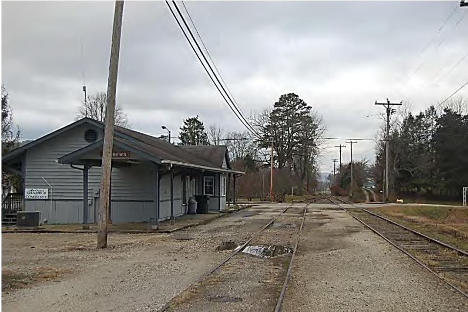
Plate 1. Murphy Branch, Looking West from Andrews Depot, Showing Station Track (Left) and Main Track.
