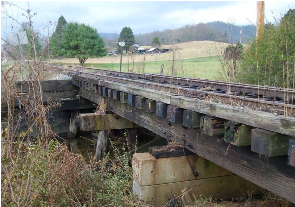
Plate 9. Murphy Branch, Railroad Bridge at Mile Post 3, Marble Vicinity, Looking West.
