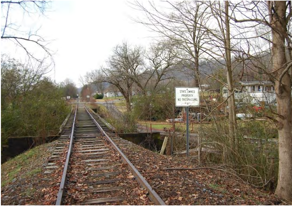
Plate 12. Murphy Branch, Railroad Bridge, East of Bluff Road, Marble, Looking West.
