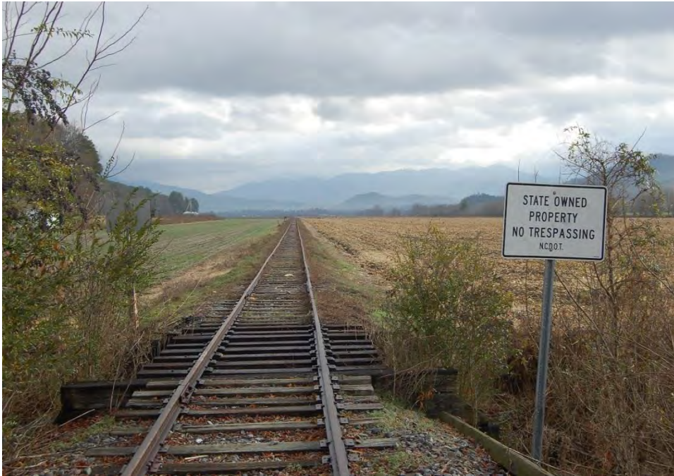
Plate 8. Murphy Branch, Railroad Bridge and Corridor, Marble Vicinity, Looking West.
