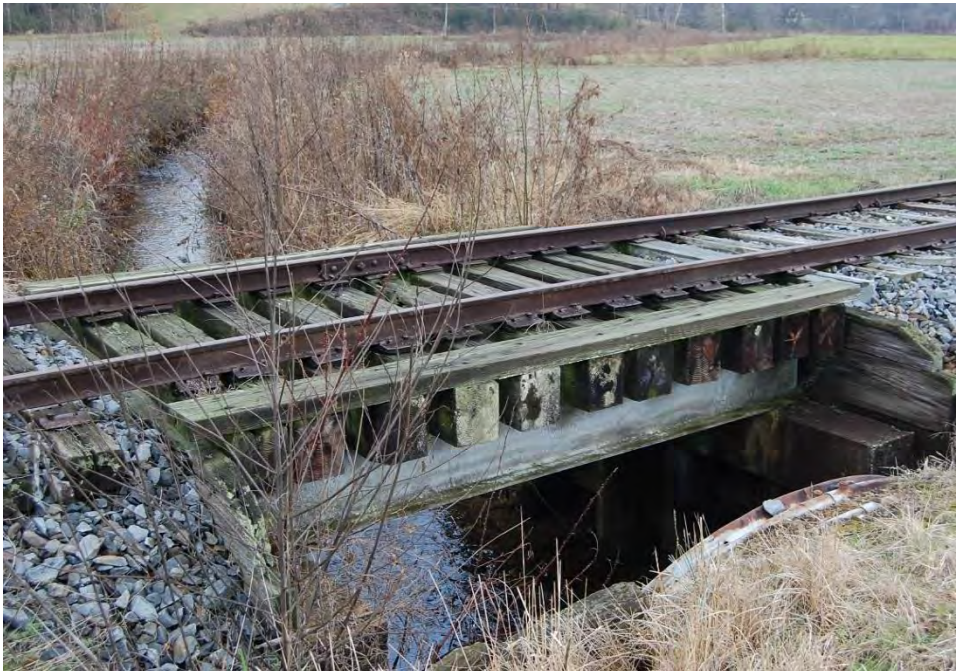
Plate 7. Murphy Branch, Railroad Bridge near Mile Post 102, Coalville Vicinity.
