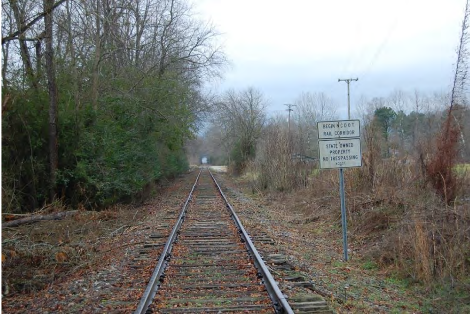
Plate 2. Murphy Branch, Rail Corridor Looking West, Andrews.
