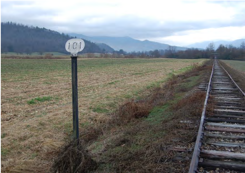
Plate 6. Murphy Branch, Mile Post 101, Looking East.
