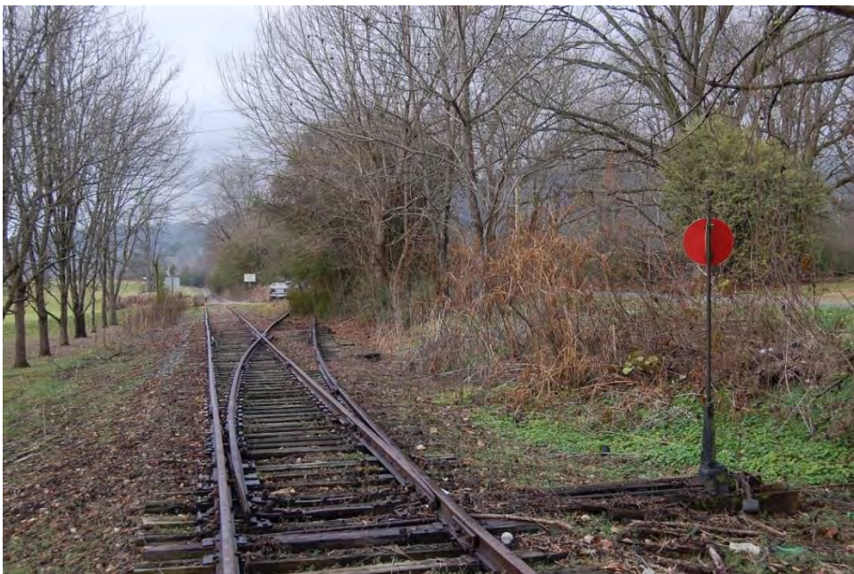
Plate 11. Murphy Branch, Switch Post at Spur Line, Marble, Looking West.
