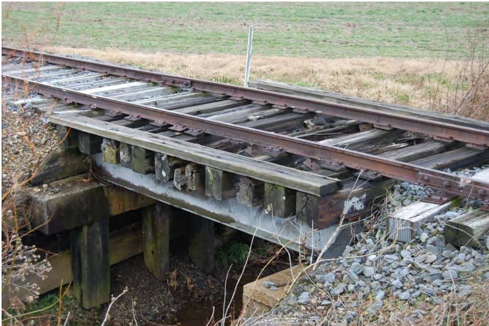
Plate 5. Murphy Branch, Railroad Bridge, Andrews-Murphy Airport.
