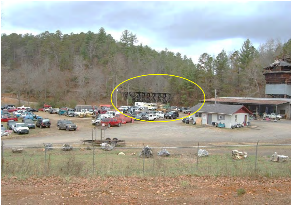
Plate 19. Murphy Branch, Railroad Bridge over Valley River (Plate 18), Looking North from Regal Street, Murphy Vicinity.
