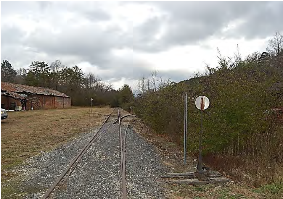
Plate 21. Murphy Branch, Rail Corridor and Switch Post near Ramsey Street, Looking West, Murphy Vicinity.
