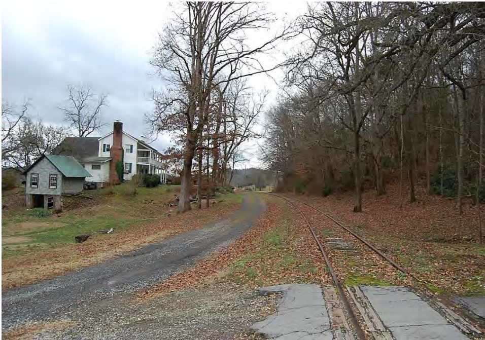
Plate 17. Murphy Branch, Rail Corridor passes circa 1850 George W. Hayes House (CE0067) (Study List 1979), Looking West, Tomotla Vicinity.
