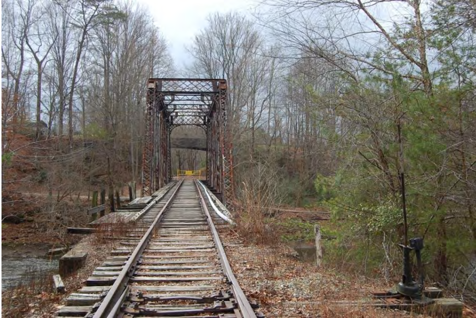
Plate 22. Murphy Branch, Pratt Truss Railroad Bridge over Valley River, Looking West, Murphy.
