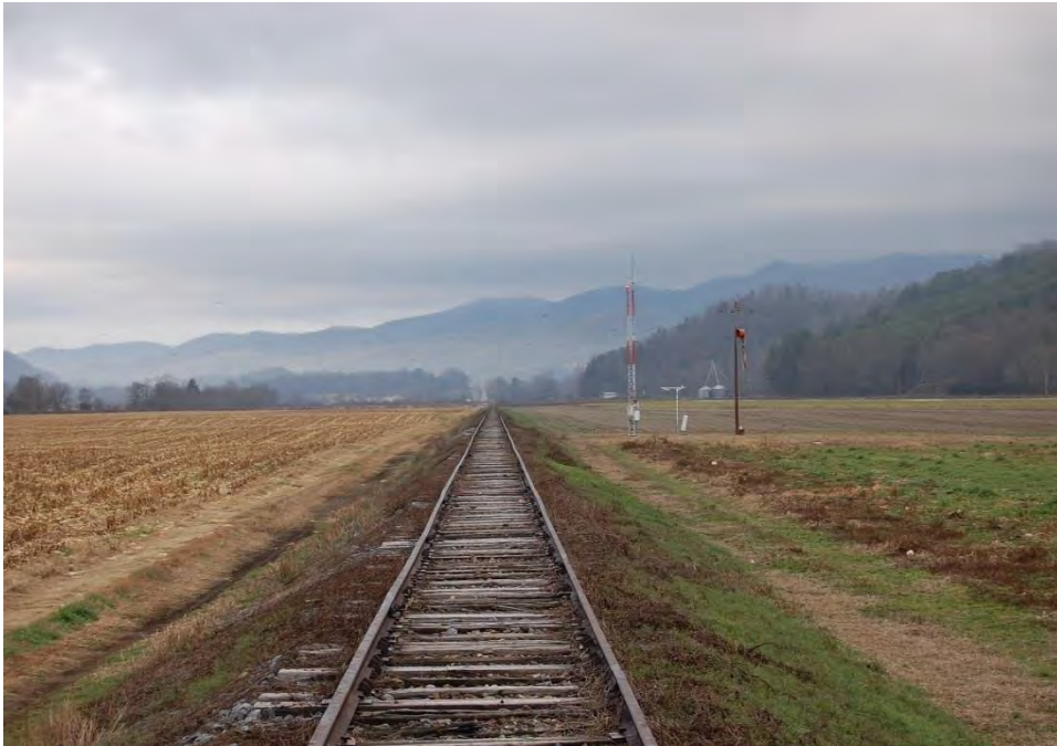
Plate 4. Murphy Branch, Rail Corridor, Andrews-Murphy Airport, Looking West.
