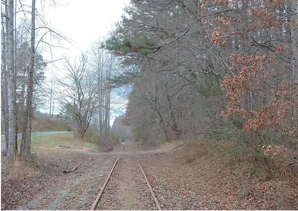
Plate 20. Murphy Branch, Rail Corridor along Ramsey Street, Looking West, Murphy Vicinity.
