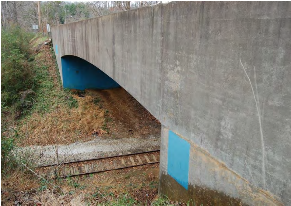
Plate 25. 1940 Reinforced Concrete, Tee Beam Highway Bridge (Plate 24).
